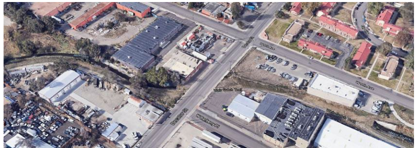
Weir Gulch Undergrounded and Inaccessible Concrete Channel – an Opportunity for Environmental Justice
